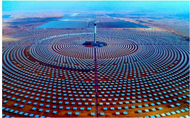
Figure 39: “Concentrated Solar Power (CSP) systems use mirrors to focus sunlight and generate electricity efficiently.
