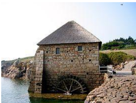
Figure 13: Tidal current mills convert the kinetic energy of tidal flows into mechanical power, historically used for grinding grain.
