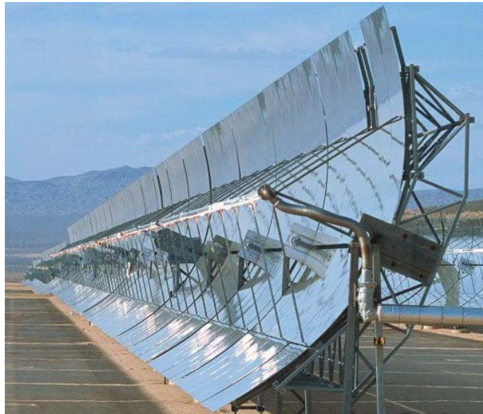
Figure 50: Parabolic trough collectors focus sunlight onto a central tube to produce high-temperature heat for electricity generation.
