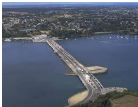
Figure 93: The Rance Tidal Power Plant in France, with a capacity of 240 MW, is one of the world's first and largest tidal energy projects, operating with a 750-meter dam.
