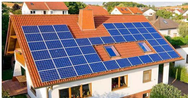
Figure 55: Domestic PV systems convert sunlight into electricity, powering homes and transferring excess energy to the grid.
